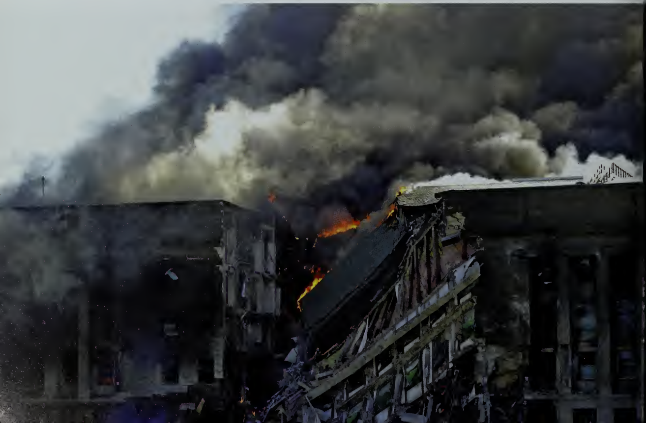
Below: Dark smoke rises from the flaming Pentagon shortly after the collapse of the E Ring.
